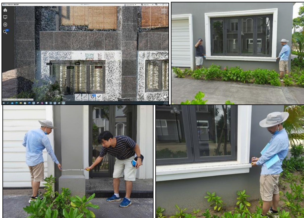
Fig 9: Measurement of Building Features on the Point Cloud and in the Field
