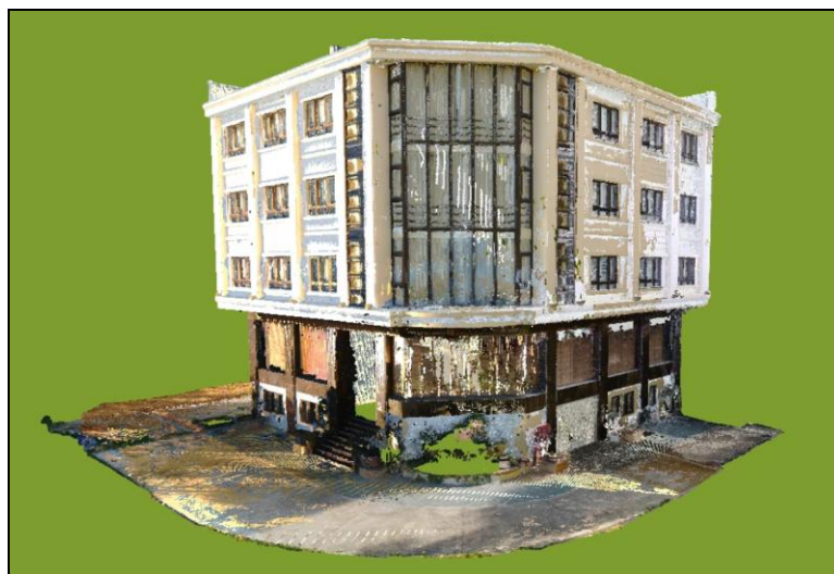
Fig 8: Fused UAV-TLS point cloud
