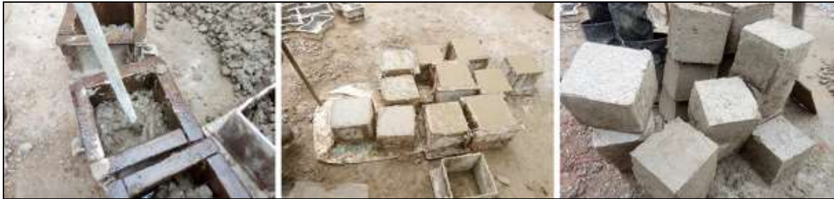
Fig 7: Production of concrete cubes
