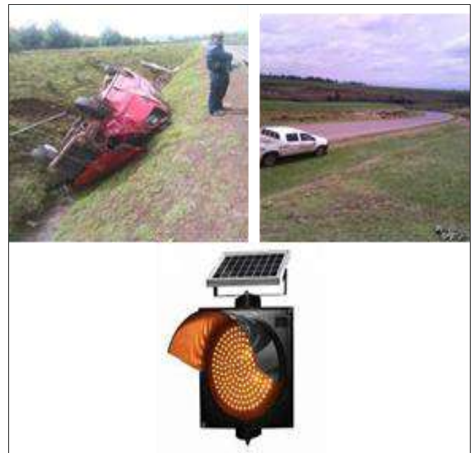
Fig 16: Hazard location after long tangent in Asella- Bekoiji in which over turning accident is dominated
