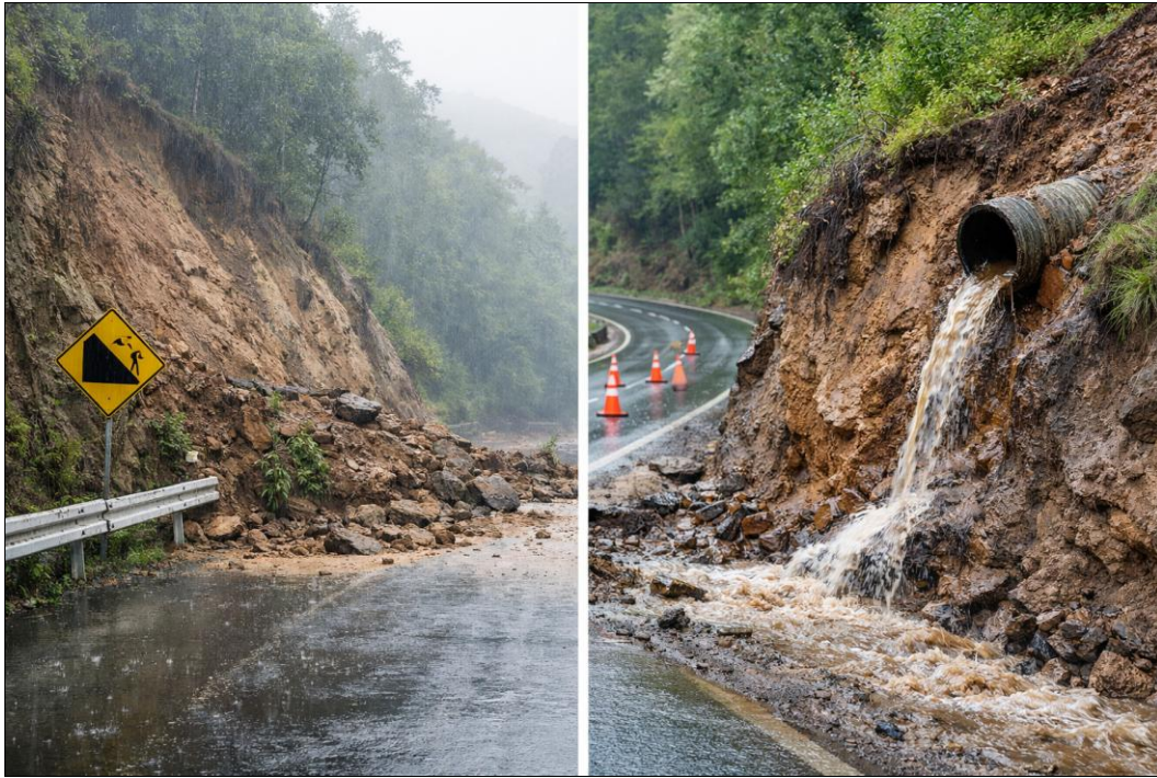
Fig 3: These images depict the impact of rainfall-induced slope instability near road cuts, with one showing debris blocking a rural road during heavy rain, and the other highlighting a steep slope failure where a ruptured drainage pipe exacerbates soil erosion.
