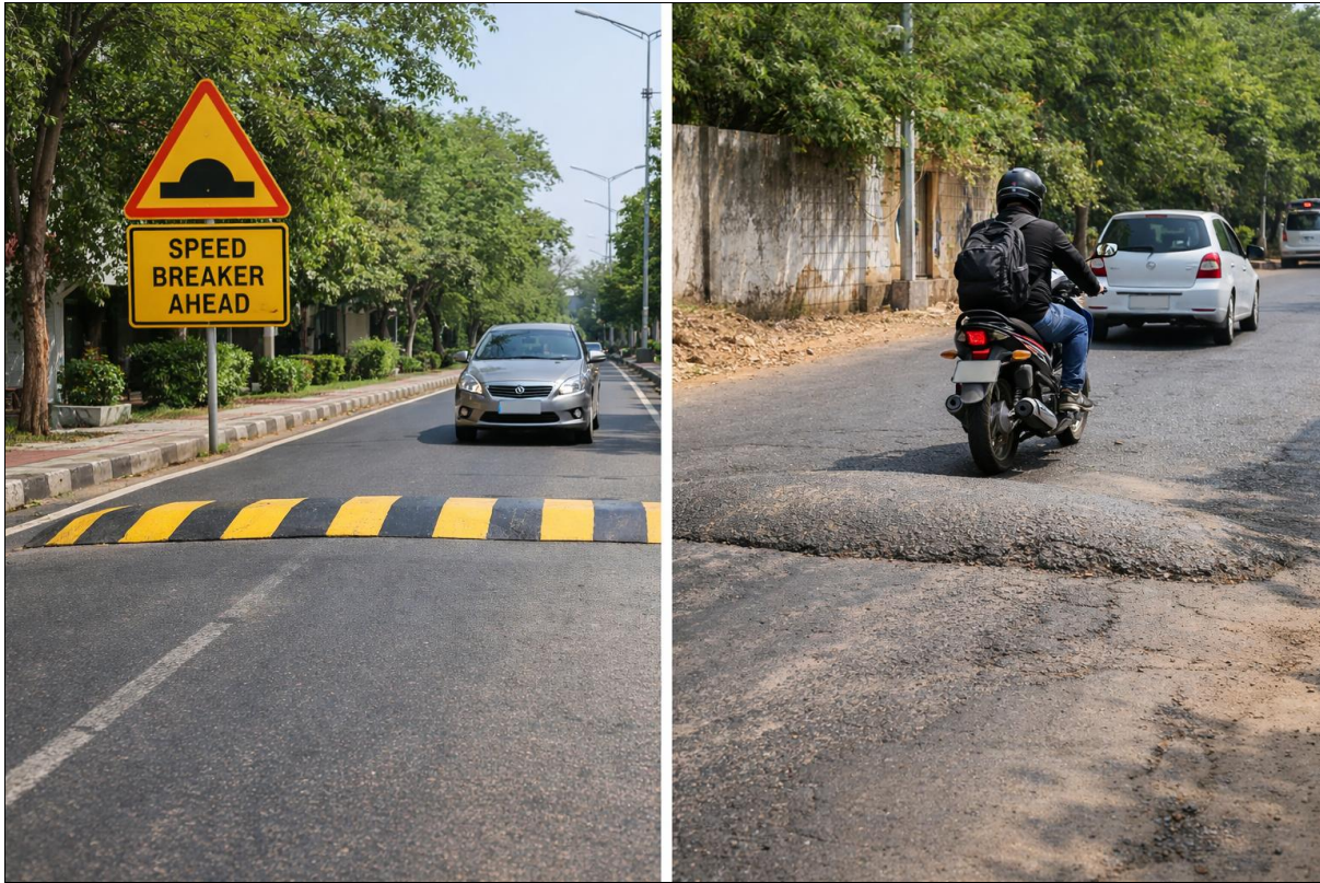
Fig 3: Two contrasting traffic calming scenarios: on the left, a well-maintained, marked speed breaker with a clear warning sign, while on the right, an unmarked, worn hump with a motorcyclist navigating through it amidst a damaged street
