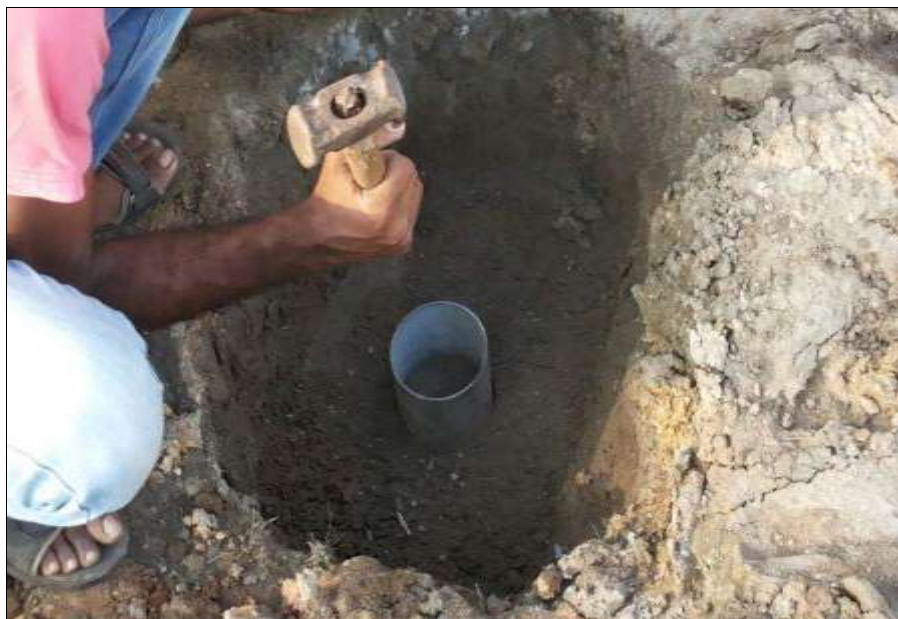
Fig 4: Typical excavation pit Building inspection
